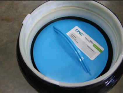
*A properly installed filter should sit below the seal area.*
